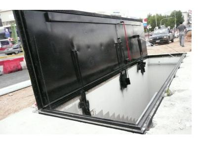
Outdoor hatches are installed to provide access to underground electromechanical networks or underground stairwells as emergency exits.
